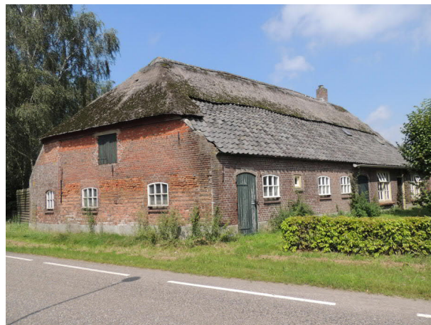
LANGGEVELBOERDERIJ IN DONK
